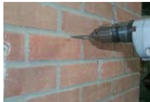
Drill pilot hole
