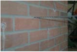
Drill pilot hole
