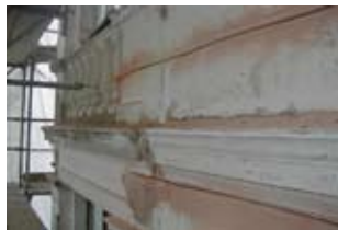
Slot clearance-flush with water
